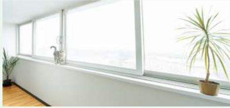
Horizontal sliding windows are a versatile option providing easy access to the outer windows of your property. The window sashes slide within the frame, making them an ideal option when limited space is available, or you need them to sit comfortably behind fitted curtains or blinds.
